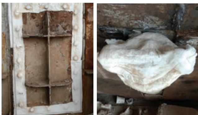
Fig 5: Conventional false air arresting methods (by ceramic paper + sodium silicate).
