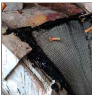
Fig 06: False Air Arresting by Arrest Master Range of Products.
