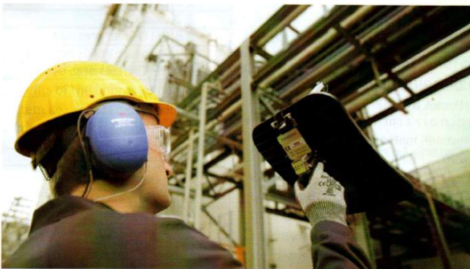
Fig. 2 False air detection by Ultrasonic Leak detector
